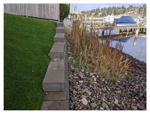
Figure 3. Detail of replacement bulkhead with turf landward and wetland vegetation with cobble/gravel waterward (12.3.20)
